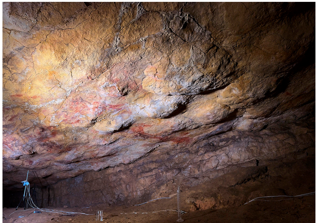
Figure 11. South area of the ceiling of the Polychrome Hall affected by carbonate concretions produced by the access of seepage water through the fracture zones.
